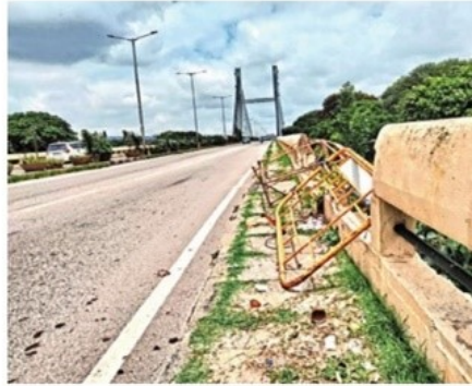
Metal barricades have been put up at the broken flyover
