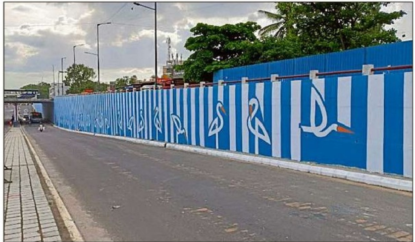
The walls of the four-lane underpass were repainted by 'The Ugly Indian' as part of a CSR project. SPECIAL ARRANGEMENT
