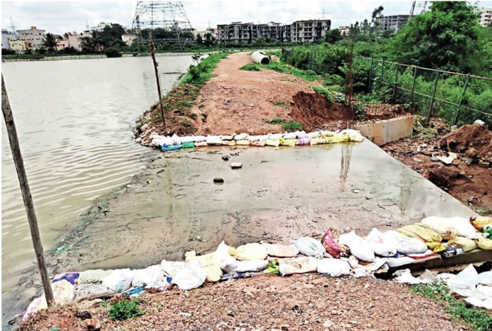
A concrete waste weir was constructed at Hoodi Lake to arrest the overflowing water, but it is ineffective
